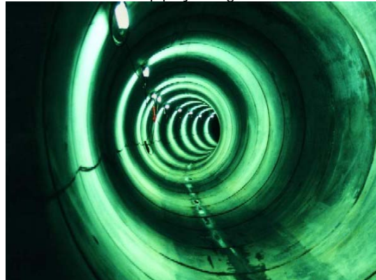
Curve pipe jacking tunnel
