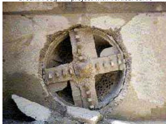
Cutting Wheel microtunnelling machine AVN1600 Breakthrough in project with vertical curve
